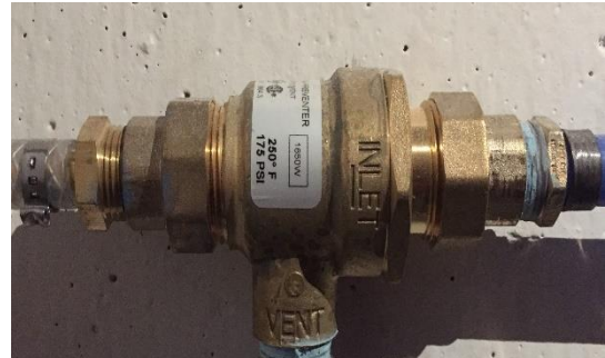
ASSE 1012: Used in place of ASSE 1022 devices except for carbonated beverage machines
